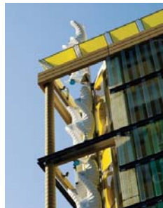
Greenway Garage, Chicago
